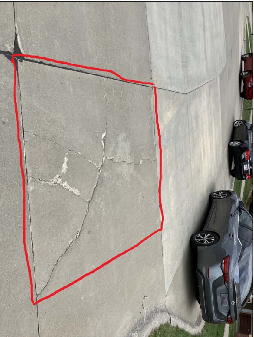
05 EAST OF BUILDING 8360: 6' X 9'
