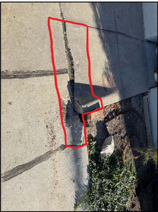
②2 CURB NORTH OF LOWER NORTH ENTRY SIZE APPROX. 4' X 2'
