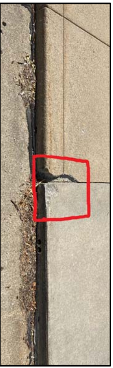
④4 CURBS AT NORTHEAST CORNER OF BLDG SIZE APPROX. 3 - 1' X 2'
