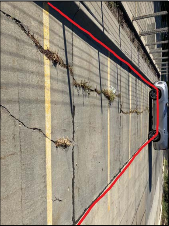
③3 UPPER LEVEL PARKING NORTH OF BLDG. SIZE APPROX. 64' X 12.5'
